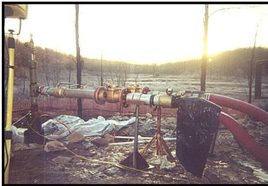
Top of well assembly for 48-hour pump test.
